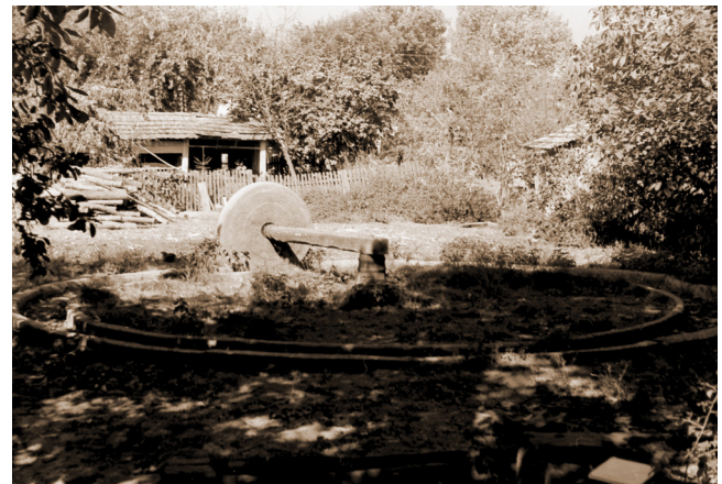
Fig. 7. Apple fermentation in Hungary: apple fruits were smashed with a special machinery similar to a mill wheel called almatörő járgány (apple-cracker capstan). (Picture is from the archive photo gallery of Janus Pannonius Museum, Pécs, Hungary).
